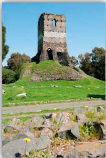
Figure 17: La Torre Selce(foto SSBAR, S. Castellani)
