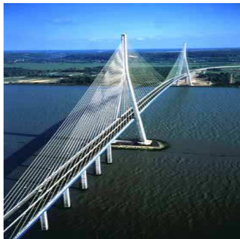
Figure -1.34- Pont de Normandie, France, 1994 (856 m) [14]
