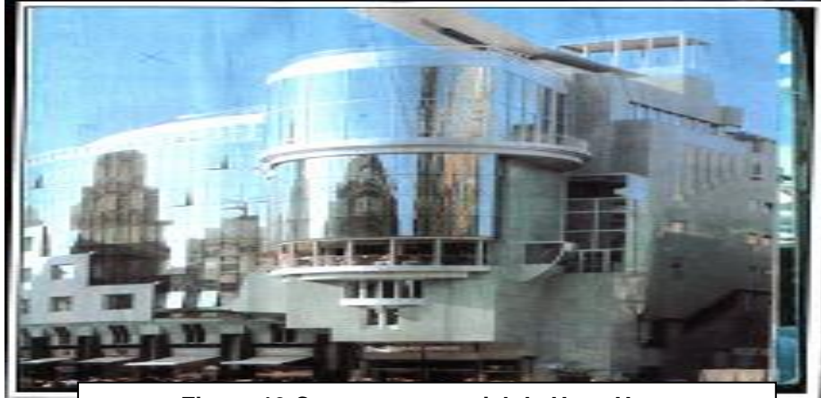
Figure 19 Centre commercial de Haas Haus
