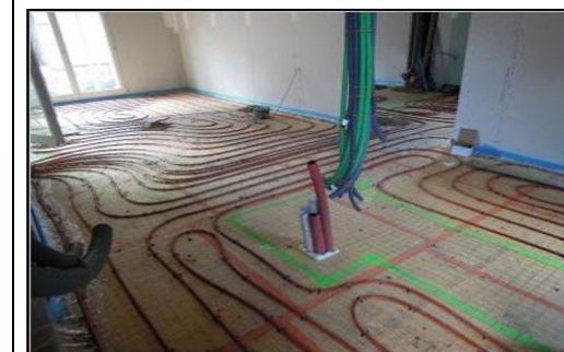
Figure II.66: Planchers chauffants Source : http://www.actuarchi.com/2011/03/26-logements-bbc-tourcoing-atelier
