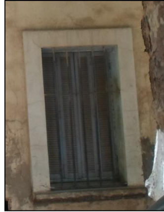
Figure III. 13 Chambranle et appui saillant
