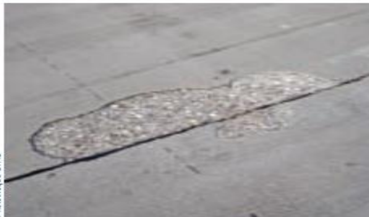
Figure I.17 : Ecaillage [5].
