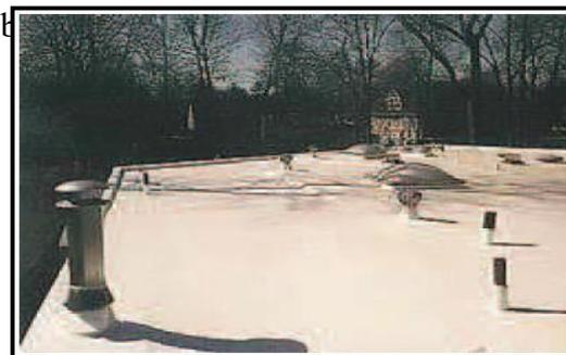
Figure 23 Membrane polyurée source (Deny & Gaumont, 2008)
