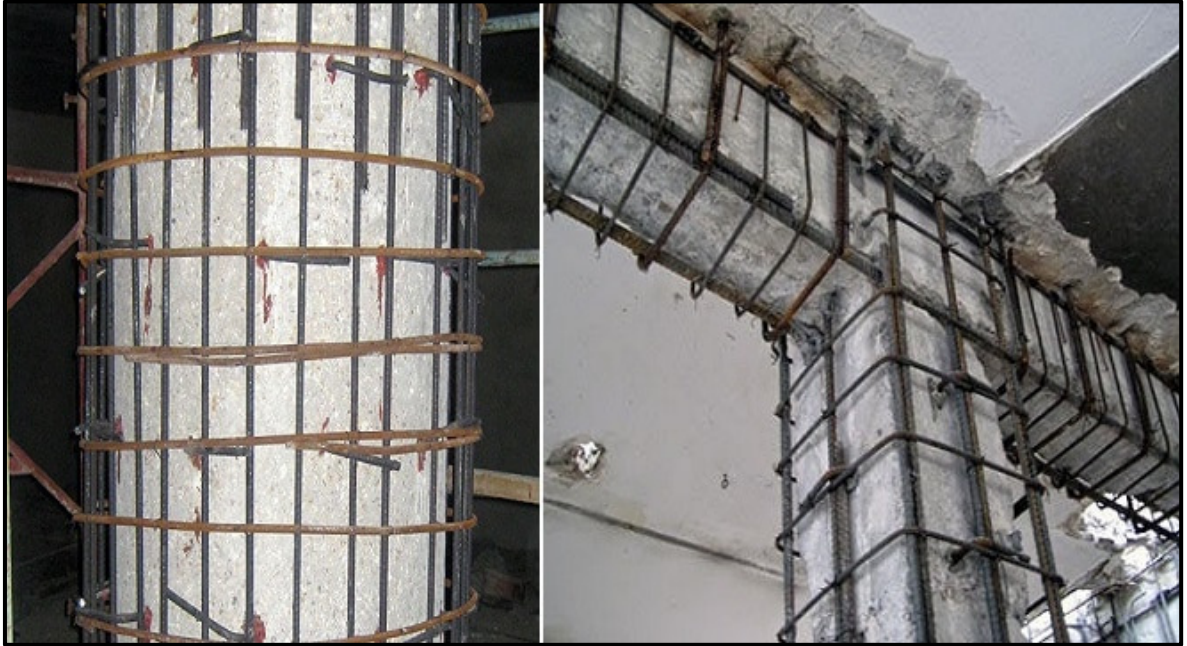
Figure II.32: Examples of column and beam jacketing.
