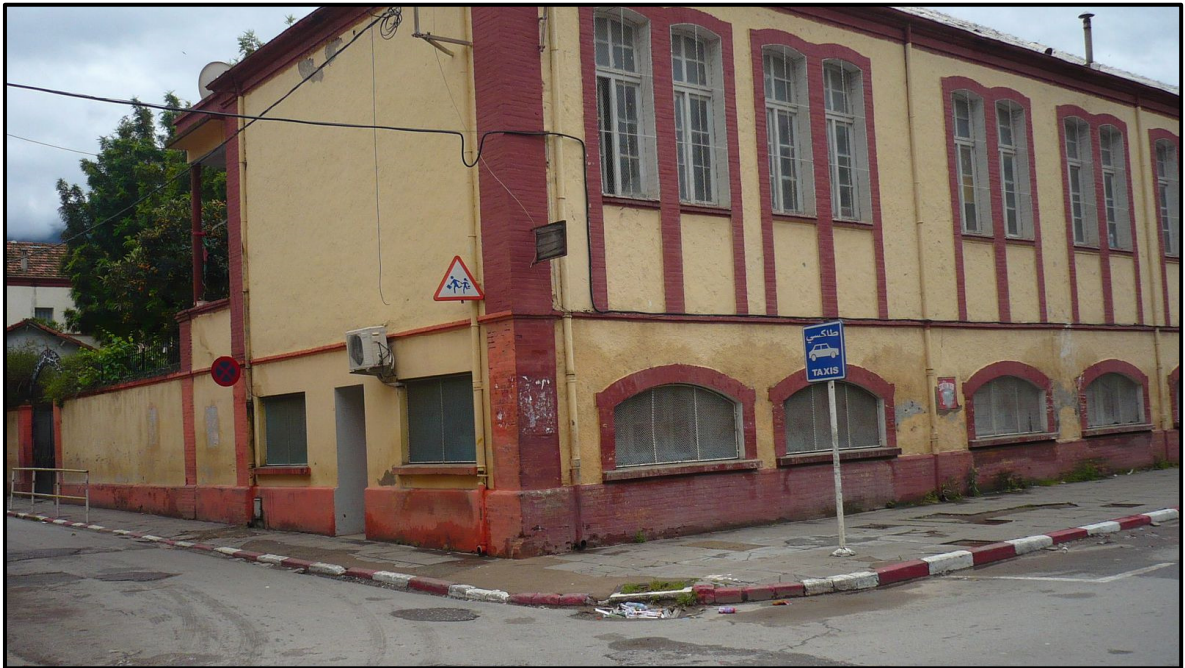
Figure II.18: Ahmed Abed primary school (Masonry building).
