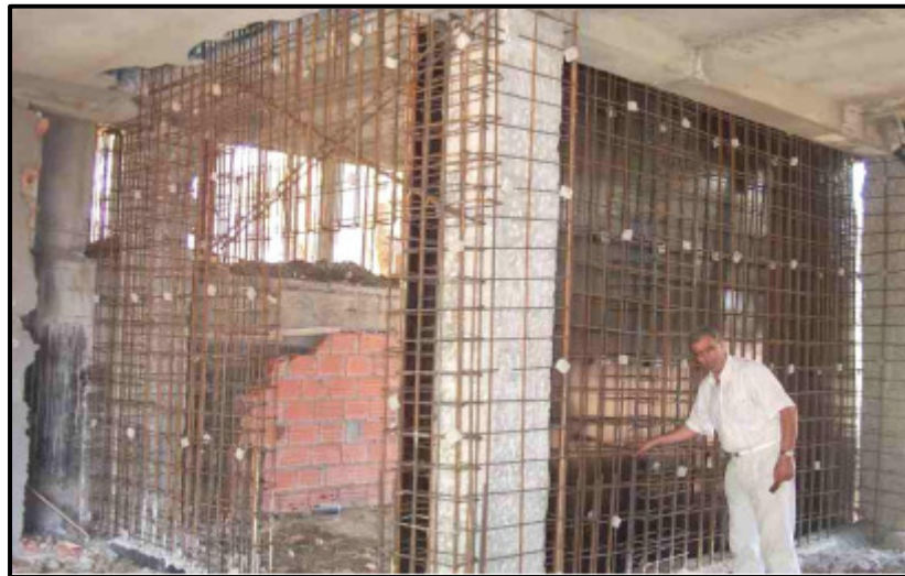
Figure II.31: Retrofitting existing building after Boumerdes earthquake by inserting shear walls.
