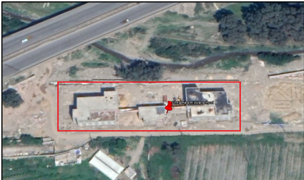
Figure III.1: Localization of the middle school under construction.
