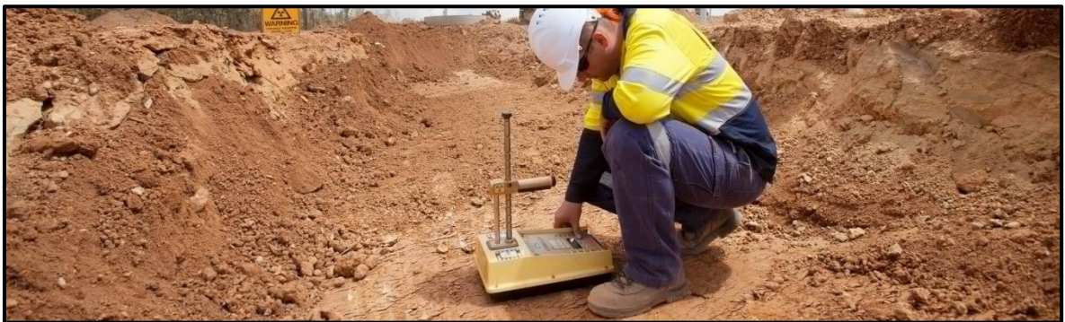
Figure II.24: Geotechnical engineer performing soil tests.
