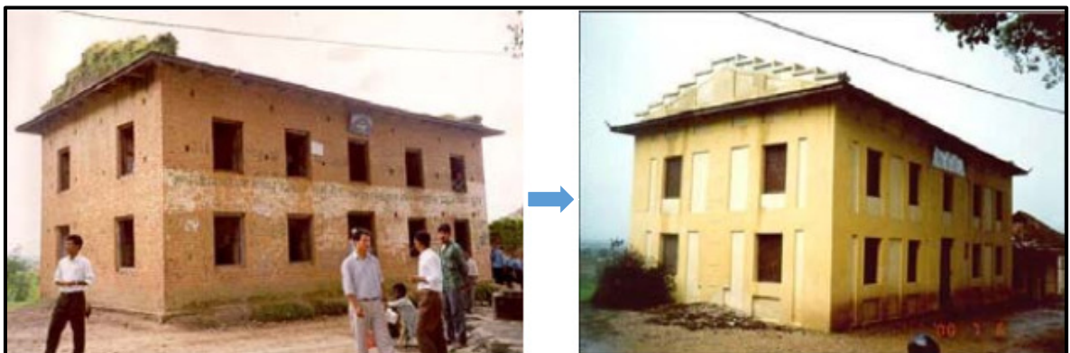
Figure II.27: Seismic retrofitting of school building in Nepal.
