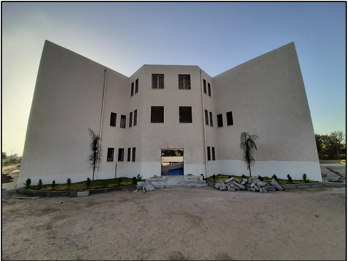
Figure II.20: A middle school under construction (RC walls system).
