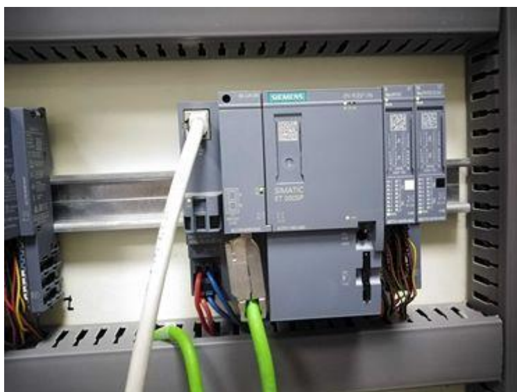
Figure 2.11. PLC ET200SP.
