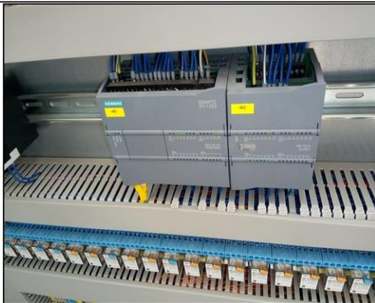
**Figure 2-4** : API siemens S7-1200 CPU 1214DC/DC/Rly.
