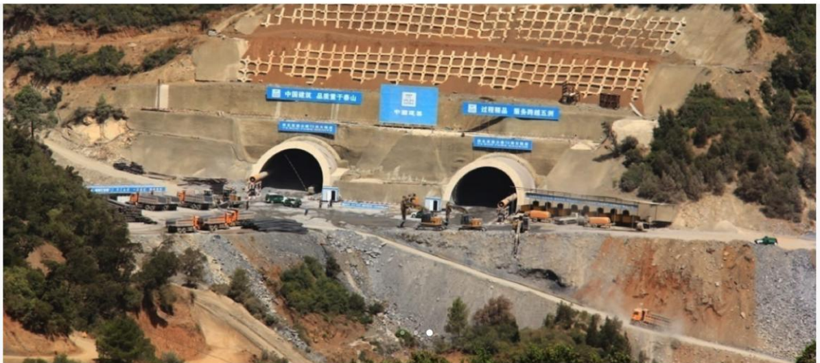
Figure I.4: Les travaux du tunnel routier d' El-hamdania.
