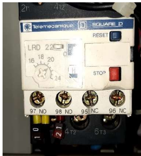
Figure II.13 Le relais thermique
