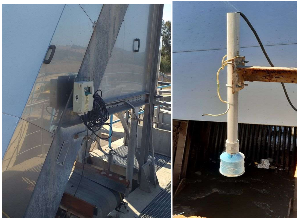
Figure II.8 Lecapteur ultrason de la station
