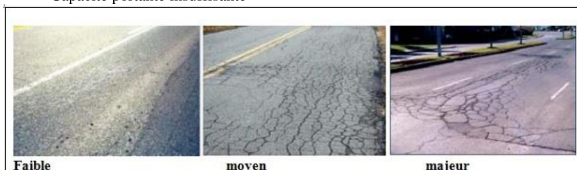
Figure 2.10: Fissures en carrelage.
