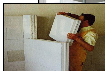
Figure 193 : La pose de siporex (Source :
