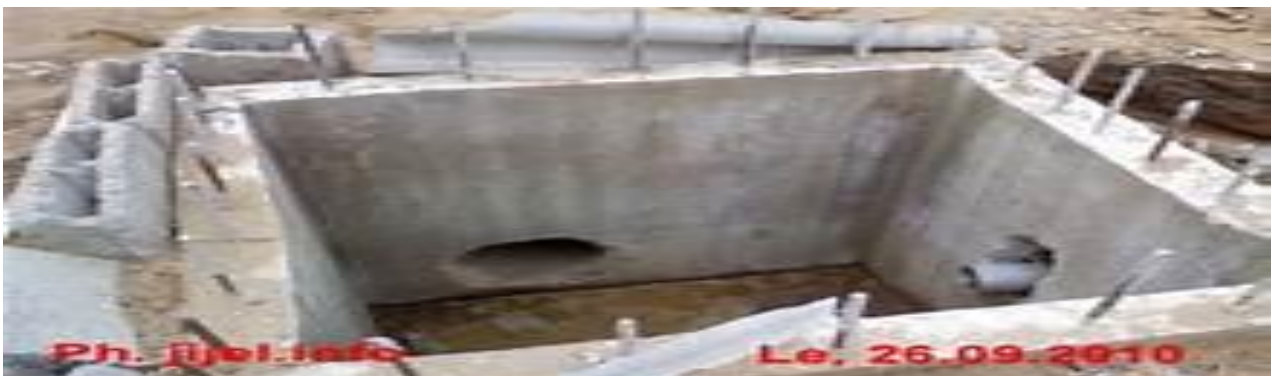
Figure VI.13. Regard de chute (source: Google image)
