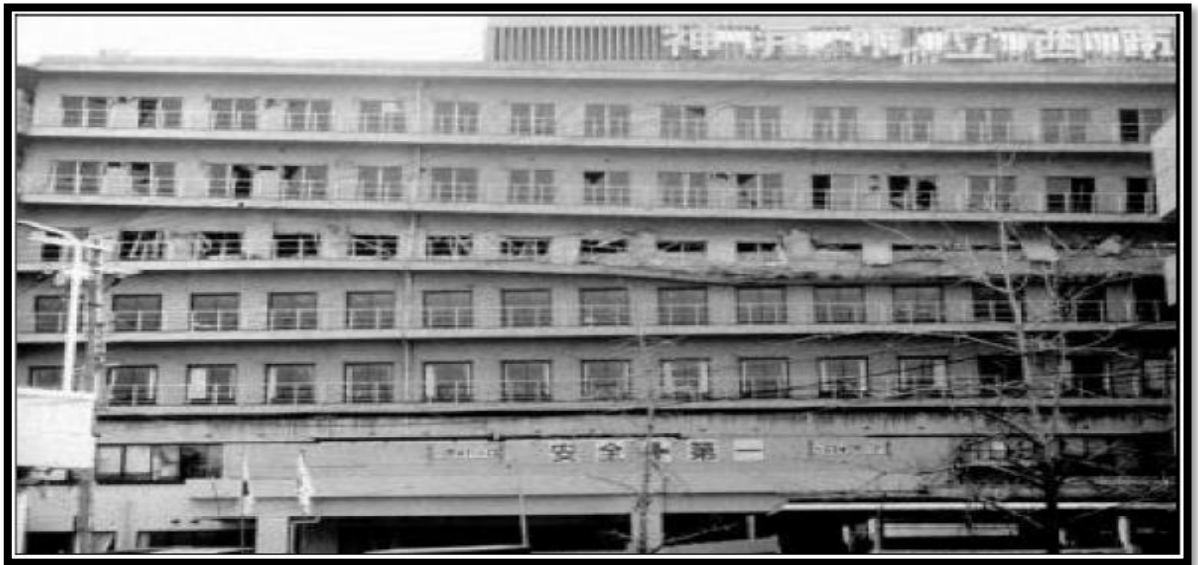
Figure 1. 2: Collapse of the fifth floor of the Municipal Hospital, Kobe, 1995. (Paho, 2000).
