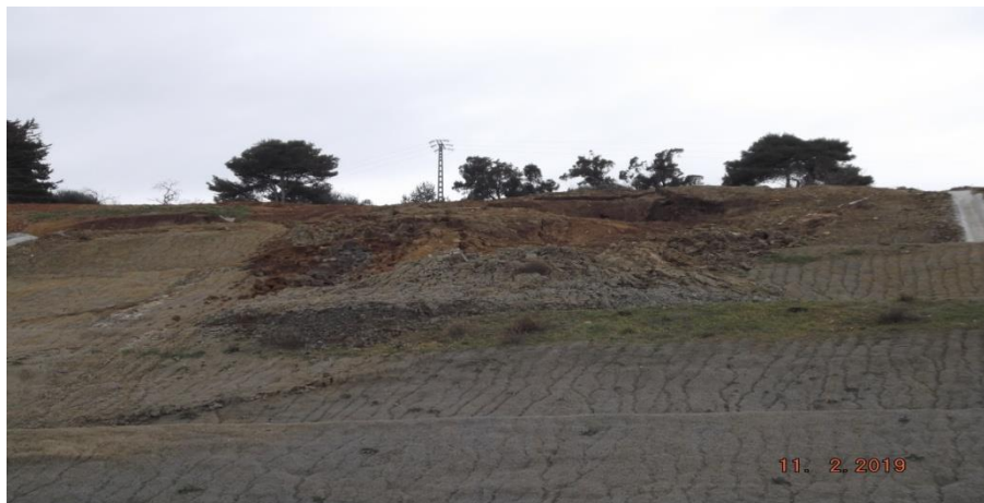
Photo II.5: Modification des pentes. [6]
