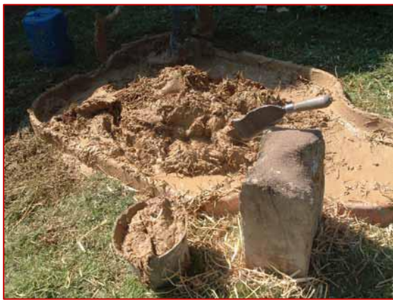
Figure 4: technique de construction de torchis
