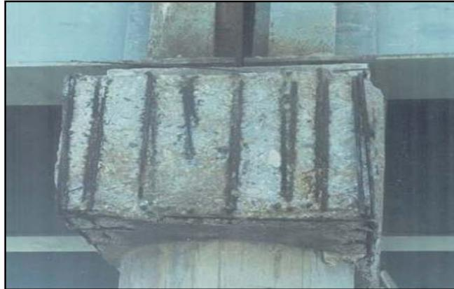
Figure I-12: Corrosion des armatures [9].
