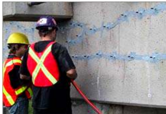
Figure I-14 : Injection de fissures [8]
