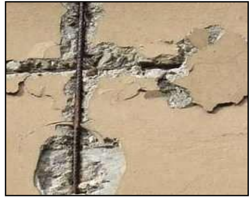
Figure 40 : La corrosion
