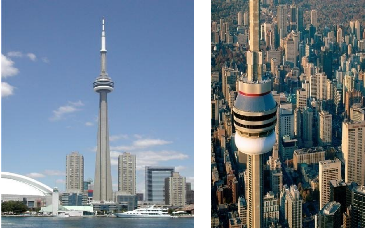
Figure 1.12 : Canadian National Tower
