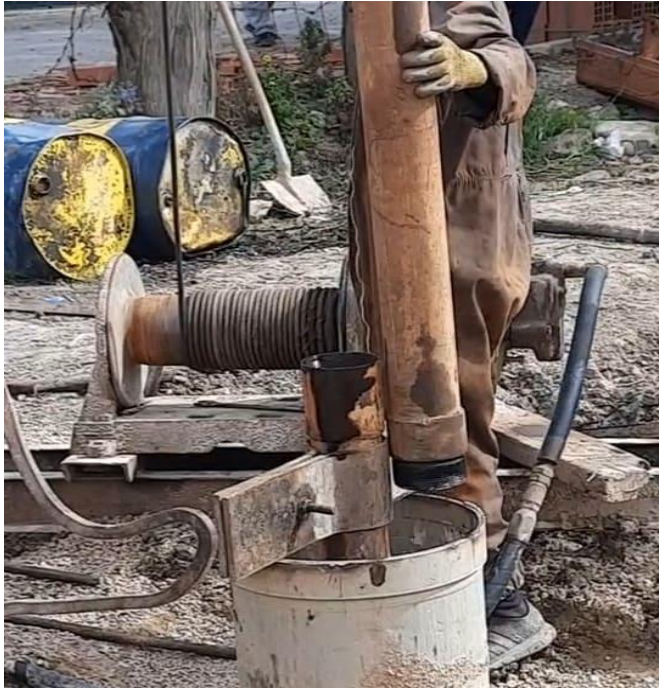
Figure 43: descente de tubage
