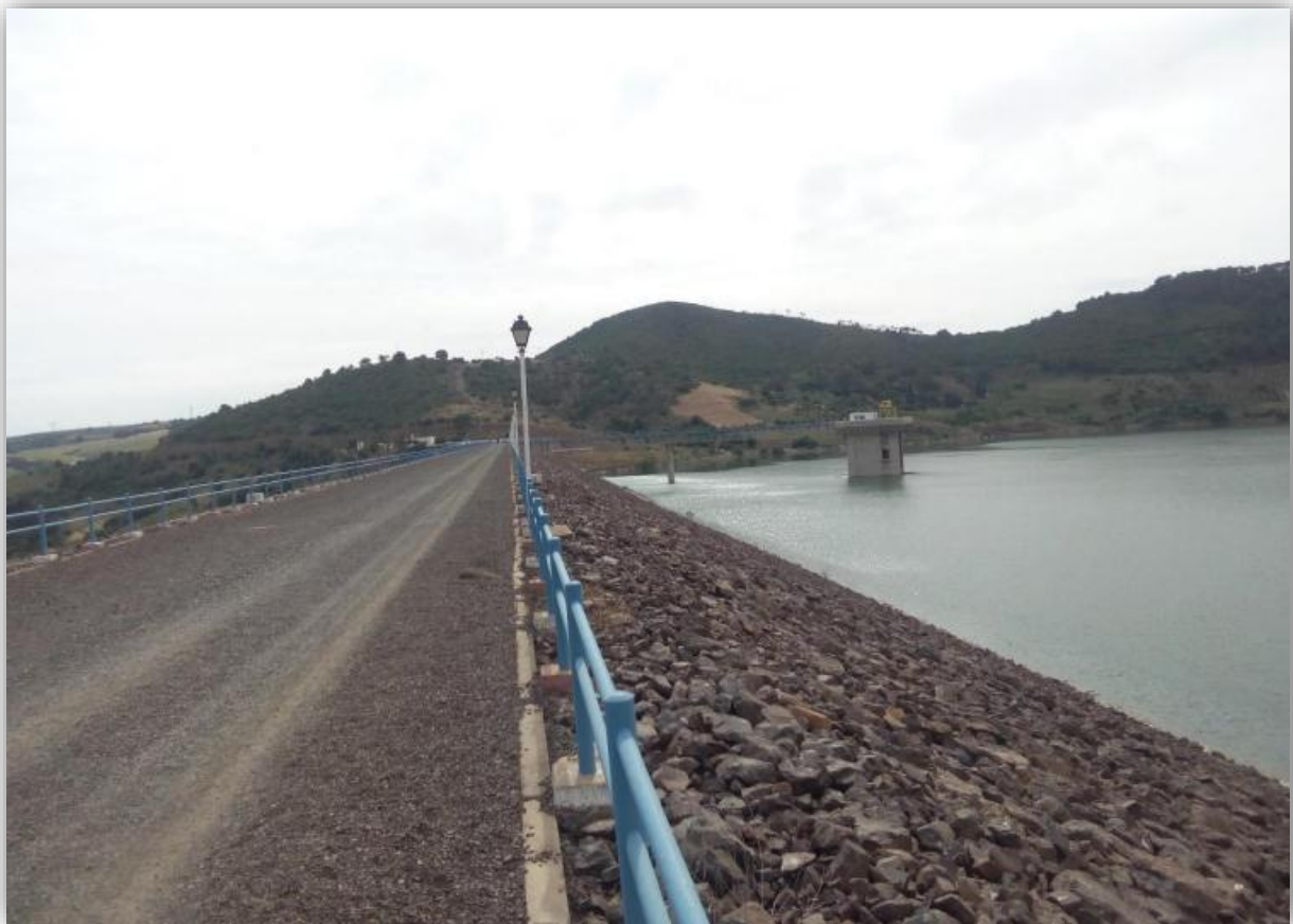
Figure 5: Barrage Boukourdane (Photo, Mai 2017).
