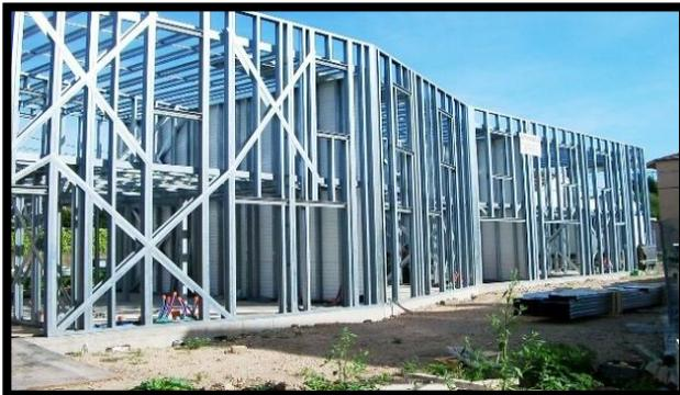
**Figure 77 .STRUCTURE METALLIQUE LEGERE**
