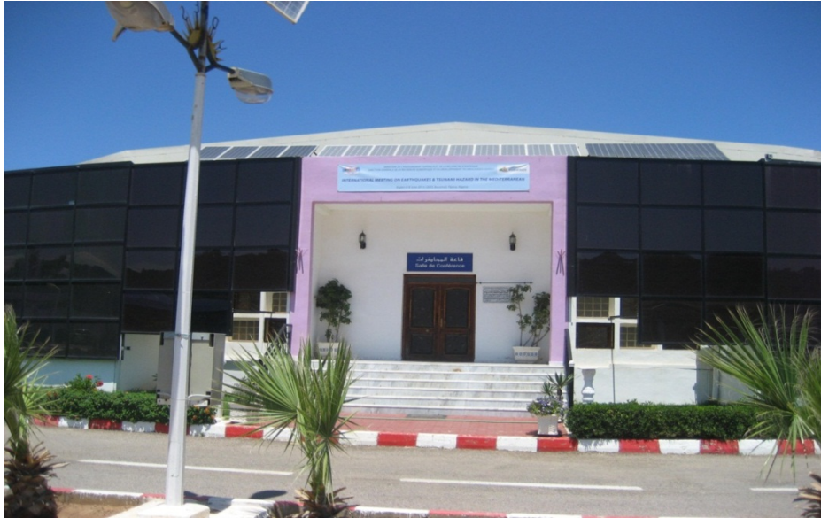
Figure 4.1- Centrale photovoltaïque de 12.5KWc de L'UDES (Bousmail)
