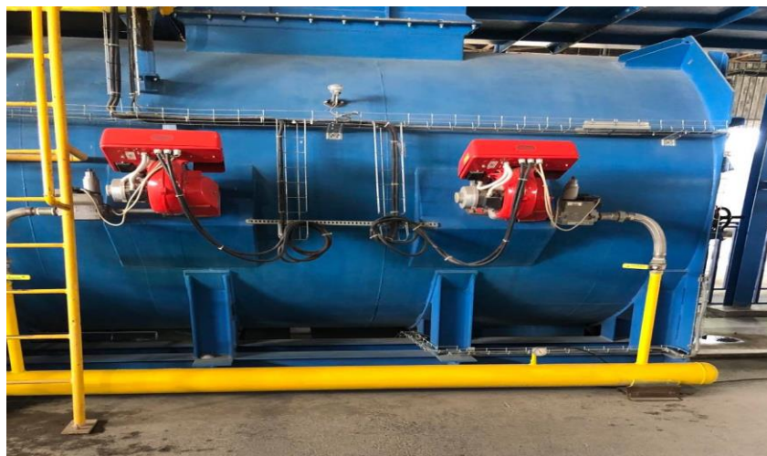
Figure III.5 : chambre de combustion
