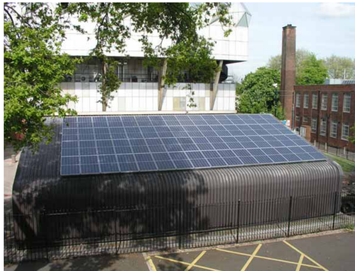
Figure 1.13: PV array under partial shadow caused by a tree [25].
