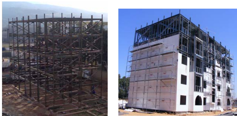
Figure 1: Typical cold formed steel frame of wall panel
