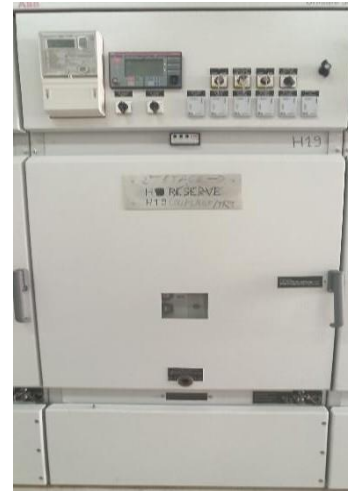
Figure 4. 11: Cellule de couplage
