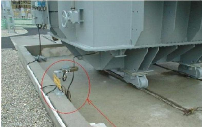
Figure 2.8 Protection masse cuve [29]
