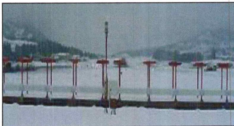
Figure 1.6: Antenne Localizer
