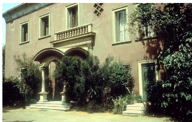
FIGURE 16 1 MONASTIRLI HOUSE GIZA, EGYPT SOURCE: HTTPS://ARCHNET.ORG
