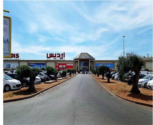
Figure(III.9) : Centre commercial ARDIS (par Google image)
