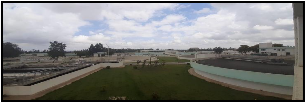
Figure 4 : Station d'épuration de Beni Mered (photo originale, 2021)
