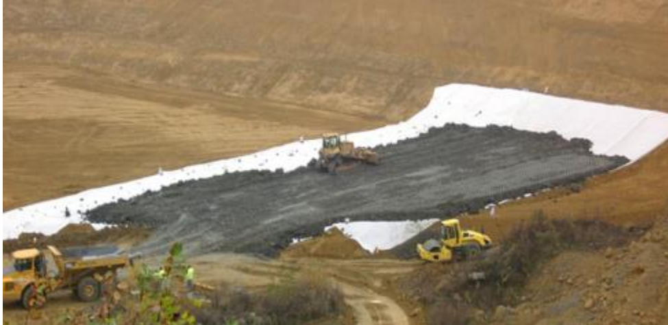
Figure II.2 : Géotextile de renforcement
