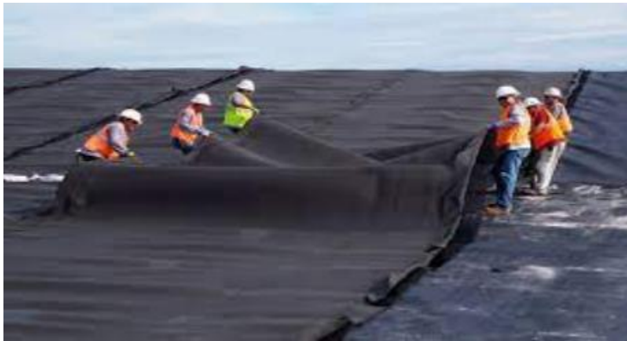
Figure II.6 : Application géo membranes
