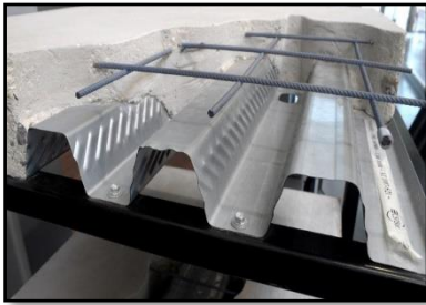
Figure 95 : Plancher collaborant
