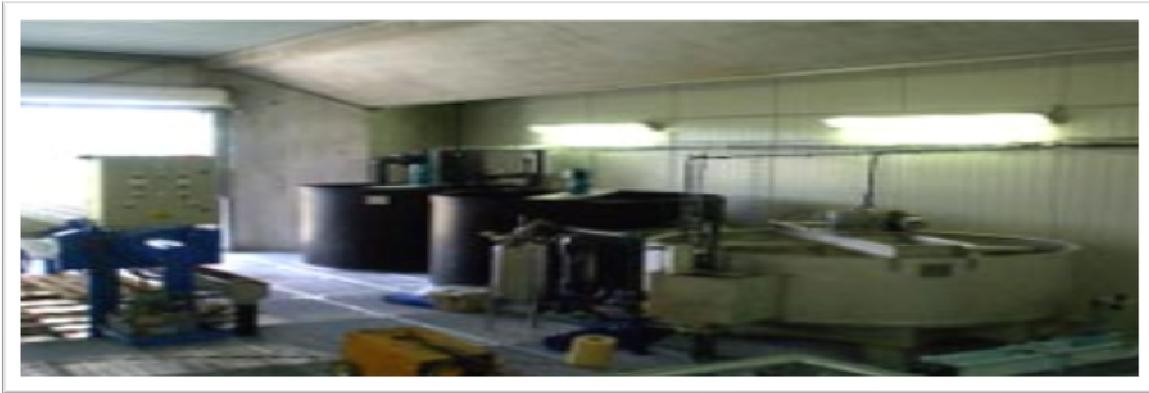
**Figure IV.5 :** Cuves de coagulation-Floculation
