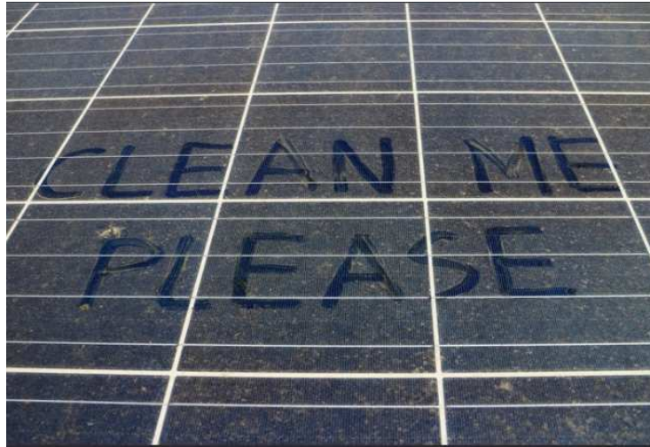
Figure 1.2. Soiling on a PV Generator.
