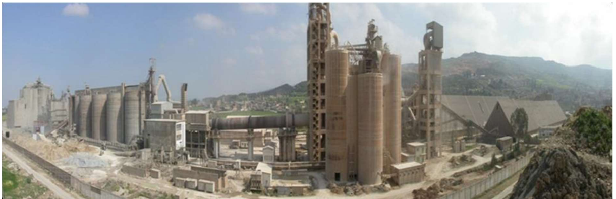
Figure 2. 3: Image of the Clinker production line of SCMI (Google Earth)
