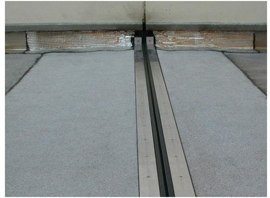
Figure 84: Joint de rupture en aluminium.
