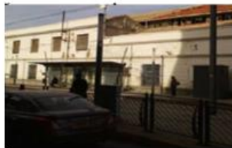
4 Station le Lycée
