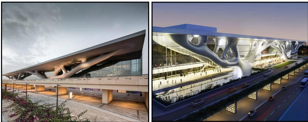
Figure 21: Qatar national convention center. Source : www.archdaily.com
