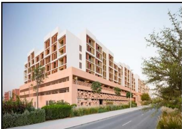
Figure 4.15: Masdar city Etihad eco-residence. source : https://www.multiplex.global/masdar-citys-
