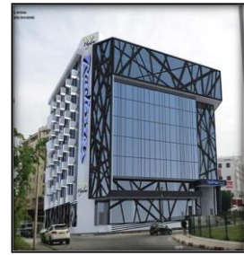
Figure 89: Radisson Blue hôtel Hydra Alger https://fr.trip.com/hotels/hydra-hotel-detail-23095144/radisson-blu-hotel-algiers-hydra/
