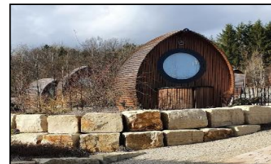
Figure 87: Bungalows. Source : Google image.
