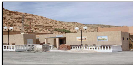
Figure 126: Station thermal Ain Ouarka. Source : Google image.
