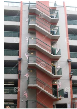
Figure 17: escalier extérieur (source: pinterest)
