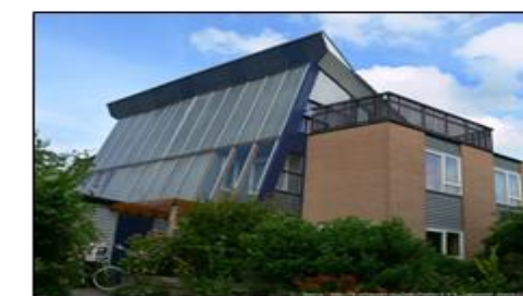
Figure 29: panneaux solaire (source: wikipedia)
