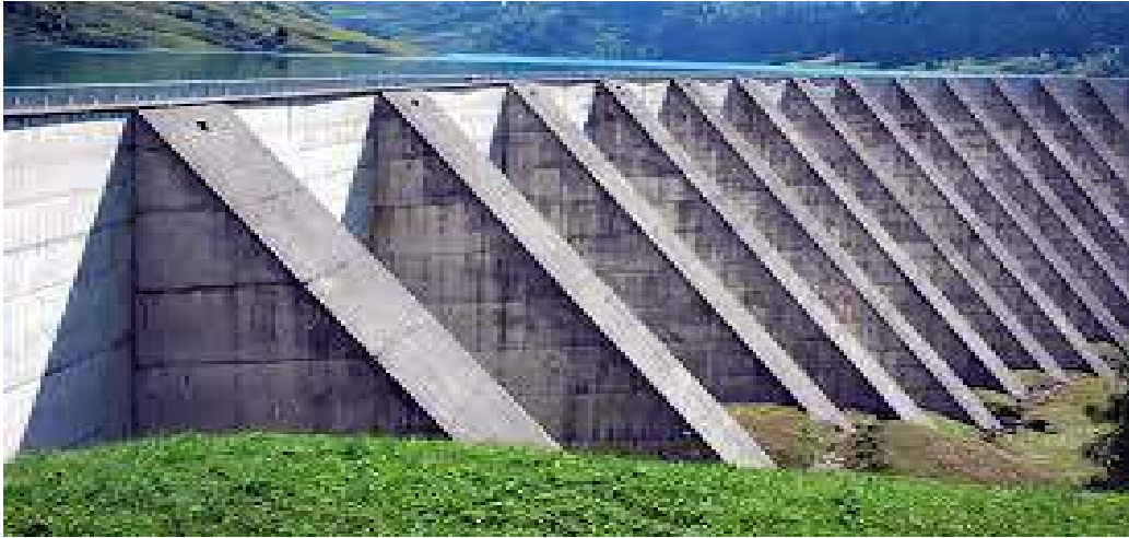
Figure I.2 : Barrage a contrefort.
