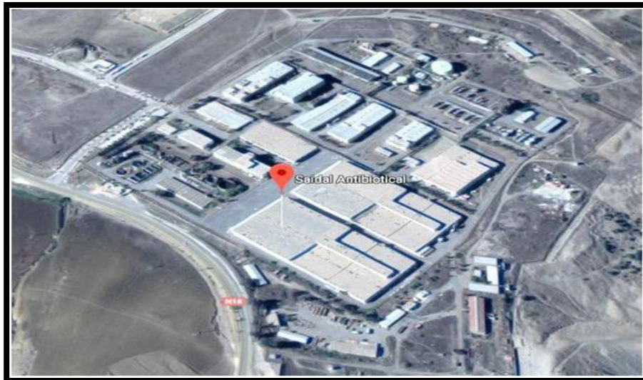
Figure I.3 : Photos satellite du complexe SAIDAL [1]
