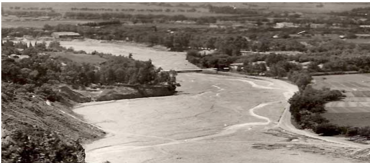
Figure XIII.13 inondation de oued Sidi el kébir [15]
